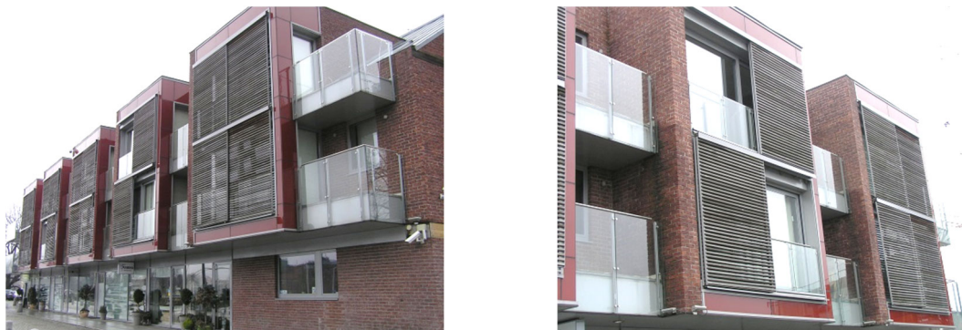
Figure 3. The sliding wooden components of the adaptive facade of the housing block in Wrocław, Poland (image: A. Krstić-Furundžić 2017)
