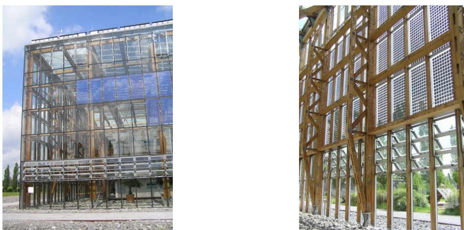
Figure 5. Facade of wooden structure with integrated PV modules, The Academy of Mont Cenis, Herne, Germany. Left: the appearance of the building, right: facade detail (image: A. Krstić-Furundžić, 2019)
