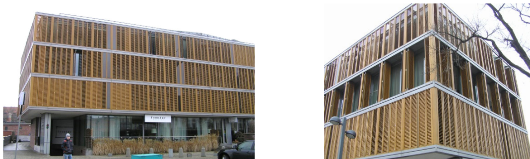
Figure 2. Vertical folding/sliding wooden components of the adaptive facade of the housing block in Wrocław, Poland (image: A. Krstić-Furundžić 2017)
