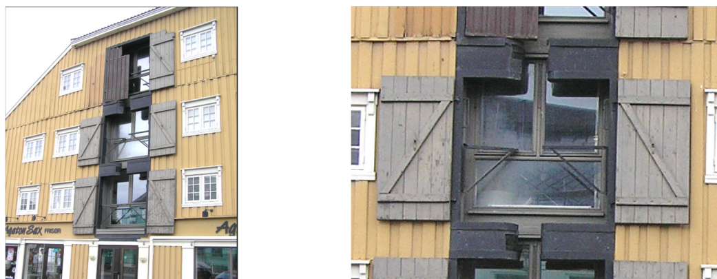
Figure 4. Panels made of solid boards as wind protection (rotate along the vertical side axis), Trondheim, Norway. Left: the appearance of the building, right: facade detail (image: A. Krstić-Furundžić 2006)
