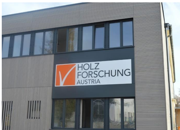
Figure 2: Silver grey semi-transparent coating that will be replaced by natural greying.
