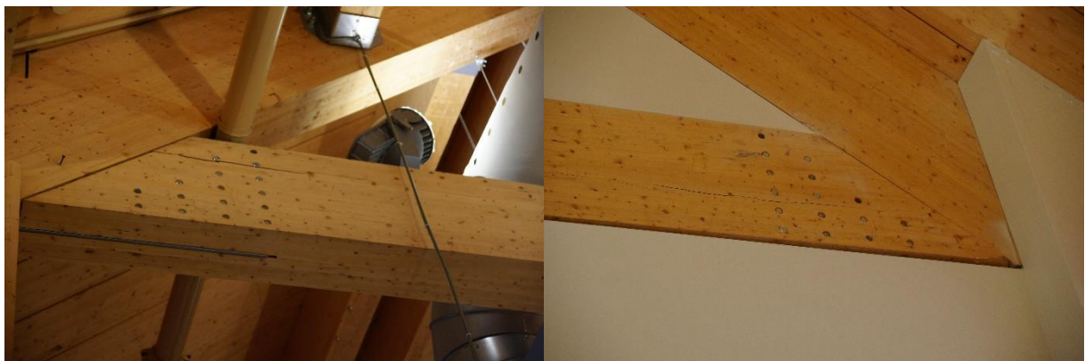
Figure 1: Cracks in the area of connections due to restraining effects
