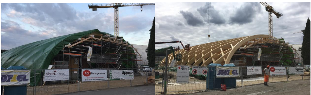
Figure 2: Efficient protection during night and weekend or rain event; removing of the protection during the working times (Swatch building, Biel/Bienne, Switzerland, Source: B. Franke)
